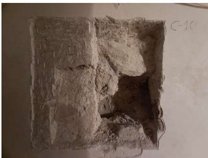
Vista general forro (1003)
